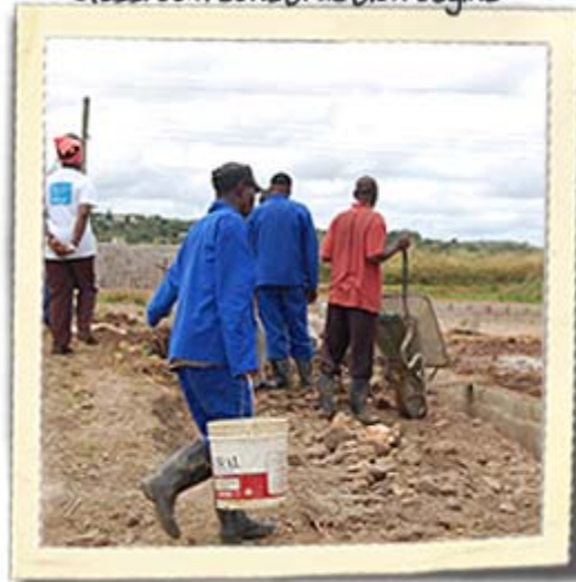
classroom construction begins!
